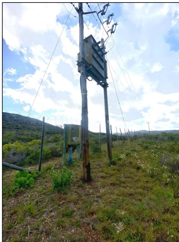
Figure 15. Electrical H pole on Plateau Road which was highlighted for re-greasing.
