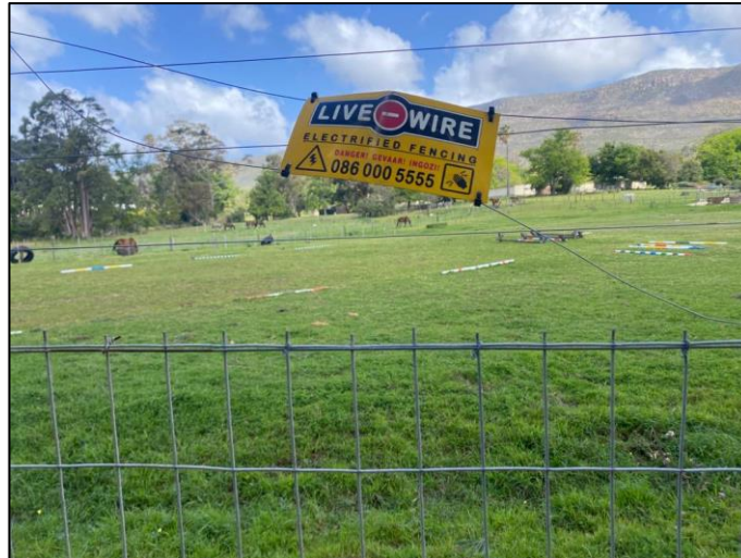
Figure 10. Broken electric fencing on the perimeter of Tokai picnic area.
